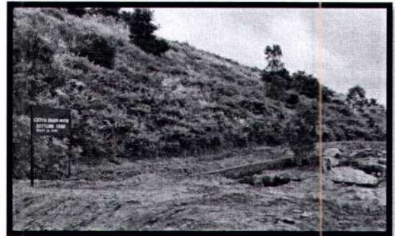
Photographs showing Toe wall and garland Drain
